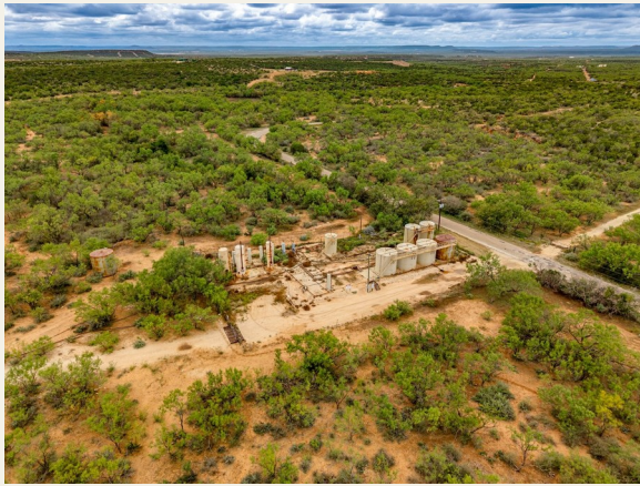
Operator tank battery and lease road.
