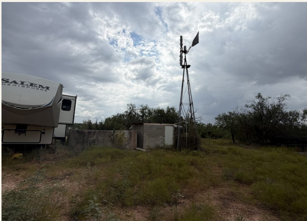
Concrete water tank and windmill. Photographed October 15, 2026.
