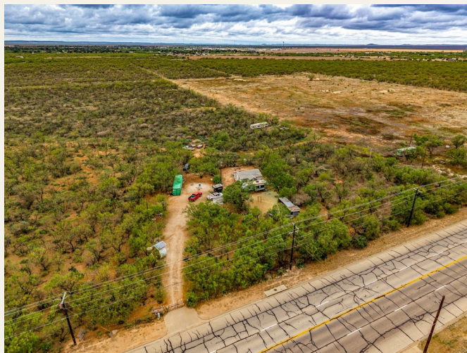
SH 208 frontage, drive and power line
